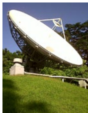
SBC05 Vertex 11m C-Band ABS-6 A & B Beams
