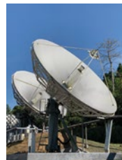
SBC10 Vertex 8.1m C-Band ABS-2 EH & GB
