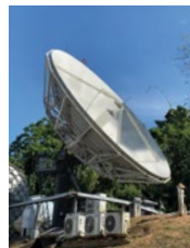
SBC09 Vertex 9m Ku-Band ABS-6 Southern
