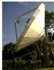
SBC07 Vertex 7.3m C-Band Backup for SBC05 ABS-6 A & B Beams
